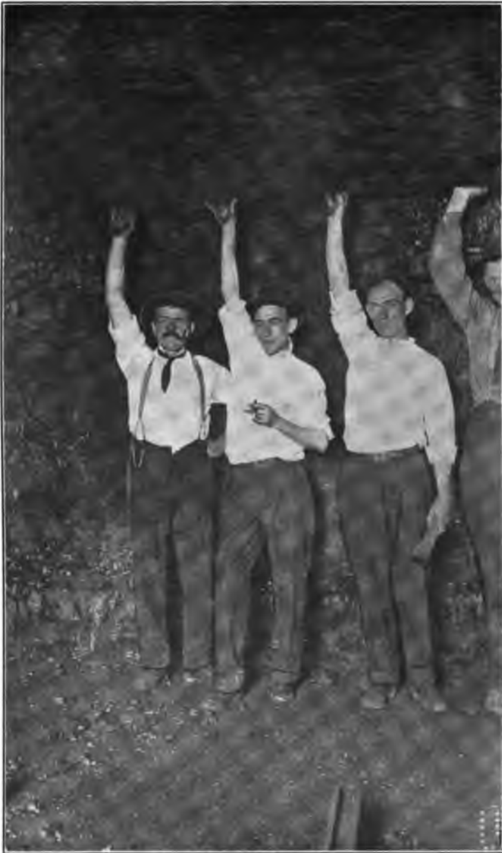
PLATE XXIV.—Winifrede Coal in mine of Anchor Coal Co., at High Coal.
